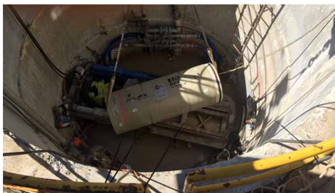
Pipe in the hydraulic jack hole.
