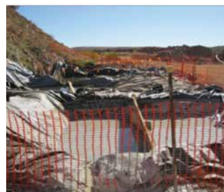
Sumps on site before using the AMC Surface SRU™.
